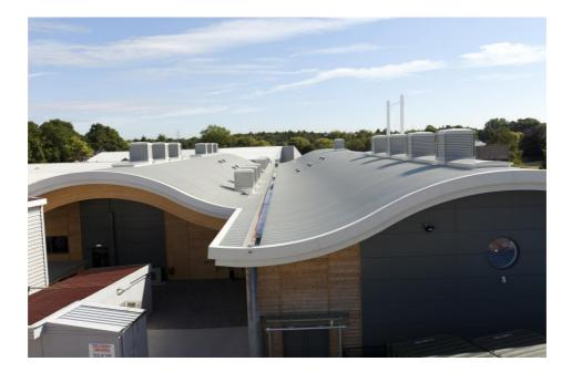
There were a number of challenges that made this project stand out; the performance of the roof being paramount. The U-value required on the roof was 0.12 W/m2K, an extremely high level of thermal insulation, which resulted in 420mm of mineral wool insulation.
