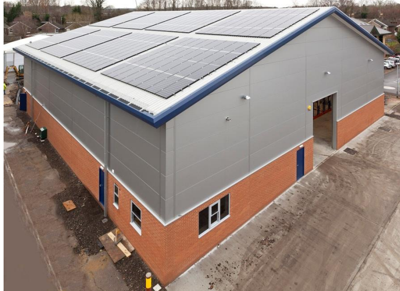
Typical example of a large scale solar PV installation: Image courtesy of CA Building Products
