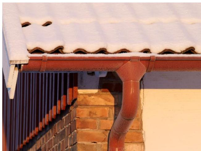
The correct position and height of the gutter needs to be carefully determined, for example, whilst a lower level fitted gutter is less susceptible to sliding snow, it could result in rainwater wind driven rainwater going between the back of the gutter/roofline which can lead to water damage to the building fabric. A gutter fitted at a higher level will alleviate this problem.
