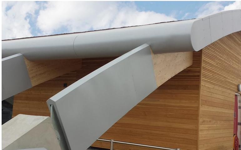
Guttercrest's range of aluminium rainwater goods and eaves solutions are incorporated into sustainable building projects on a more and more regular basis. With a long-lifespan, recyclable nature and superior aesthetic for both traditional and contemporary buildings, aluminium offers a notable option for environmentally aware building designers.
