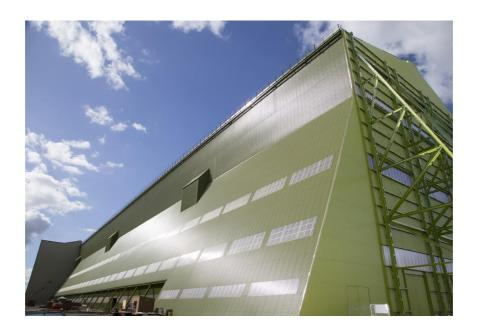
As part of the £10.5 million refurbishment on one of the largest hangars in the UK, leading rooflight manufacturer Brett Martin Daylight Systems has supplied Trilite GRP sheets. Designed to bring daylight into the Bedfordshire building, reduce the need for artificial lighting and create a more pleasant and comfortable environment for the team working on Airlander 10, the largest British aircraft that has ever been constructed.
