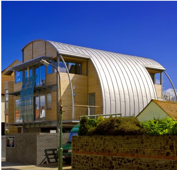
Aluminium curved roofing at Warwick Lodge Dental Centre, Essex. Image courtesy of Kalzip Limited
