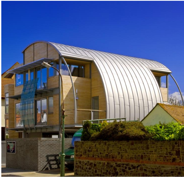
Aluminium curved roofing at Warwick Lodge Dental Centre, Essex. Image courtesy of Kalzip Limited
