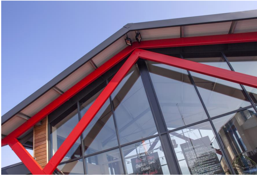
The Blyth Boathouse Restaurant which features insulated panels, flashings and purlins all manufactured and supplied by Steadmans Limited.
