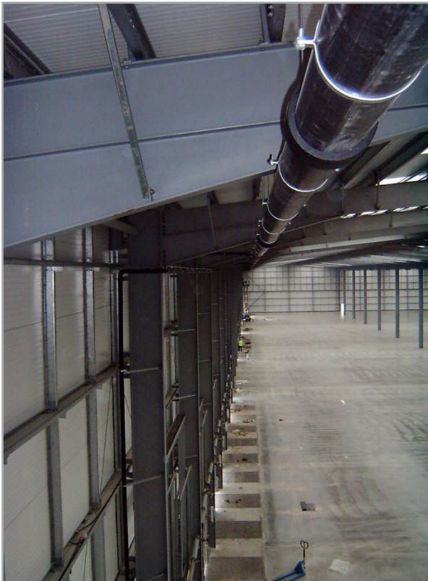
Siphonic pipework horizontal at high level
