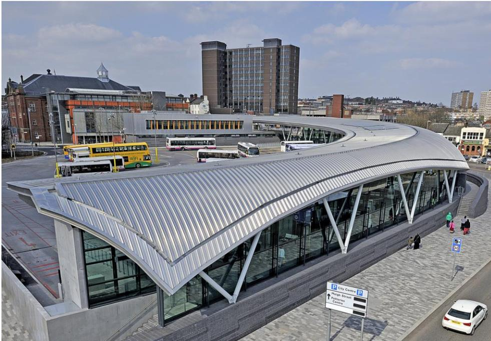
Kalzip's aluminium standing seam system was specified for the impressive new Stoke-on-Trent City Centre Bus Station by architect, Grimshaw. VINCI Construction UK was the main contractor and experienced Teamkal contractor, Lakesmere Ltd installed the Kalzip roofing system which included all the revolutionary double curvature XT profiled sheets and a bespoke Kalzip rainscreen specially designed for use on the bus drivers' accommodation block.
