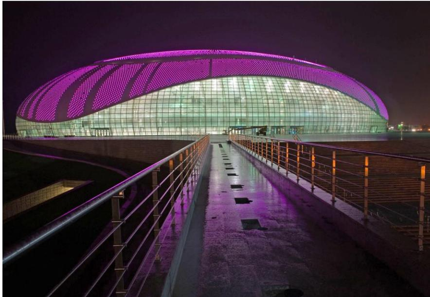
More than 22,000 square metres of tapered Kalzip aluminium standing seam sheets were used to create the weatherproof building envelope of the spectacular 12,000-seater Bolshoy Ice Dome that was used for the 2014 Winter Olympic Games at Sochi in Russia. Designed and built by SIC Mostovik, this giant domed structure has a maximum span of 193 metres, a height of 40 metres and a total surface area of nearly 32,000 square metres.
