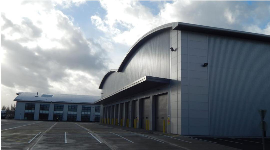
'Quantum' curved built-up metal roof and PRIME V cladding from CA Group Limited has been installed at the Blackburn Trading Estate in Heathrow as part of development work for Canmore Developments, creating a more aesthetically pleasing structure.
