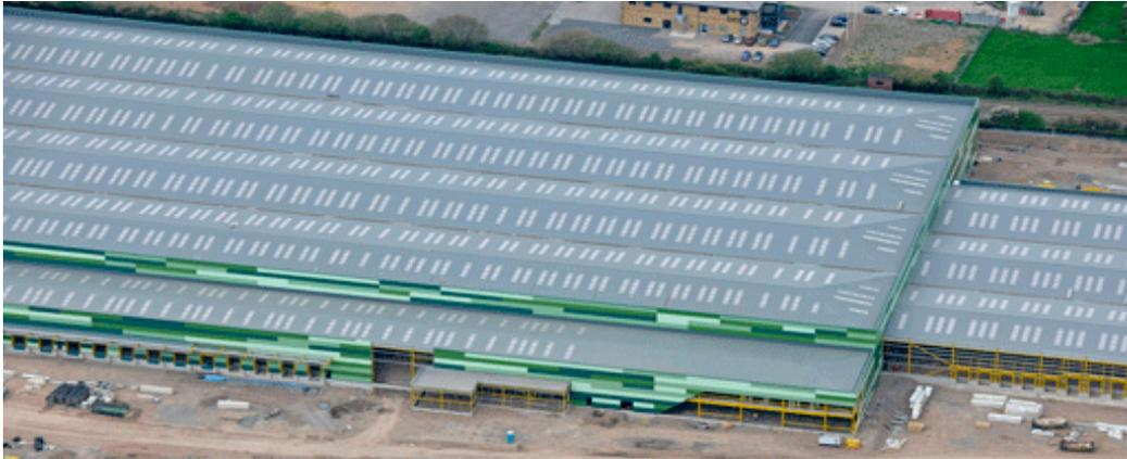
High durability, long life performance and thermal insulation were central to the specification of 10,000 square metres of Brett Martin Daylight Systems' Energysaver composite panel rooflights which have been installed in the Morrisons Regional Distribution Centre (RDC), near Bridgwater in Somerset.
