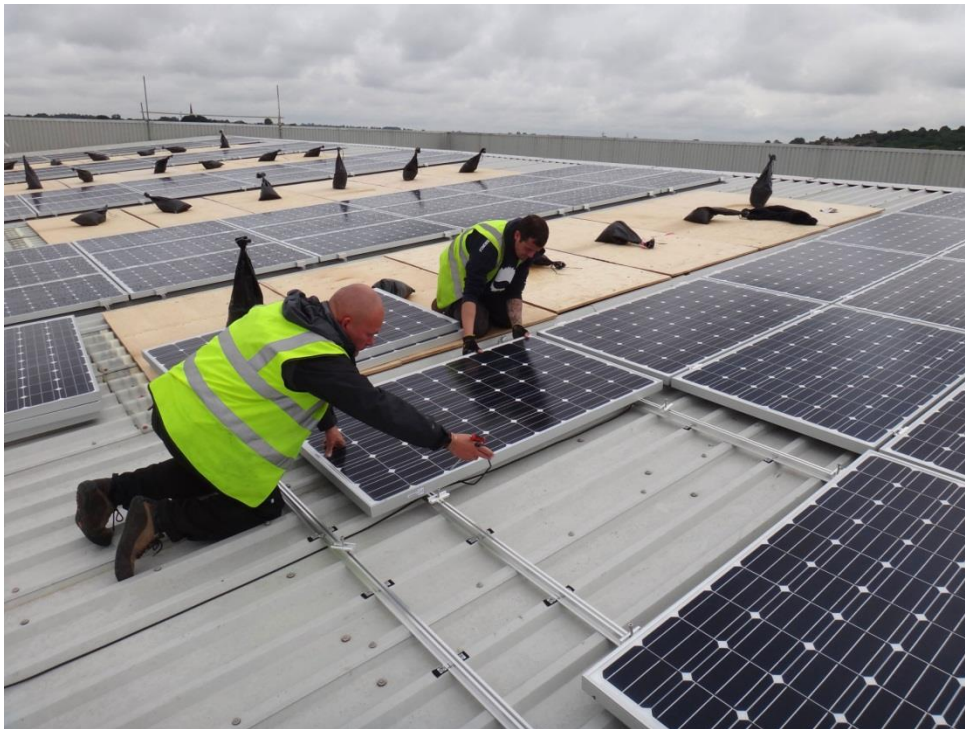
Installation of solar panels on the Hambleside Danelaw roof
