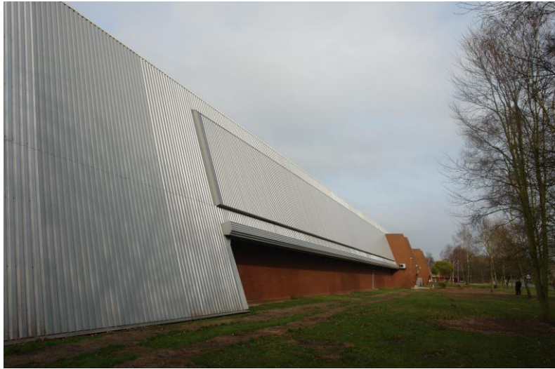
SolarWall® transpired solar collector system was used at Jaguar/Land Rover, Leamington Spa. Image courtesy of CA Building Products Limited
