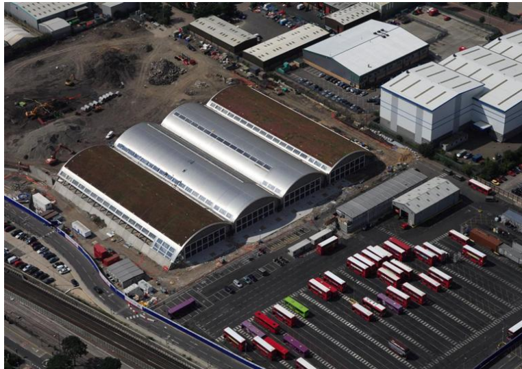
West Ham Bus Depot featuring a Kalzip Nature Roof Image courtesy of Kalzip Limited
