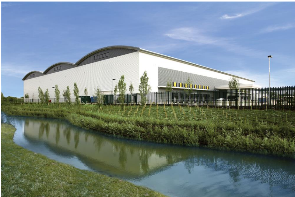
Direct Wines Warehouse, Gloucester. Image courtesy of Euroclad Limited
