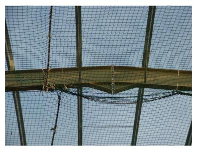
Image 2: Incomplete structural connections
