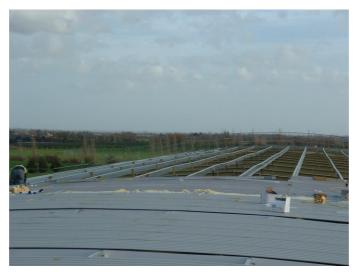
Image 1: Undulating/out of position purlin
