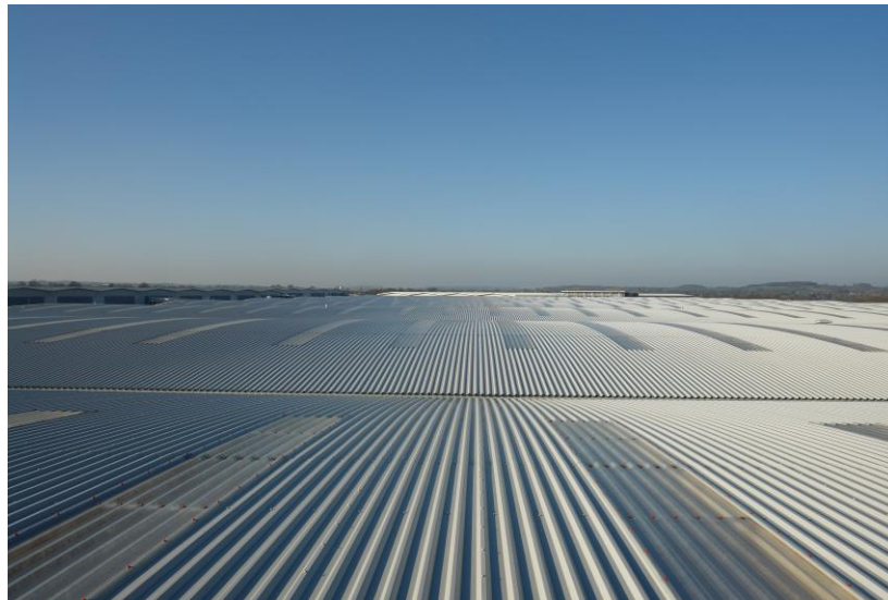
Image 3: Example of good installation and workmanship. Image courtesy of CA Group
