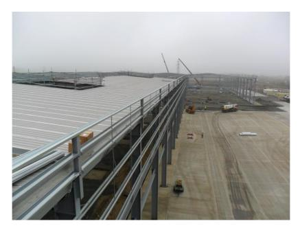
Image 4: Primary and secondary steelwork properly installed
