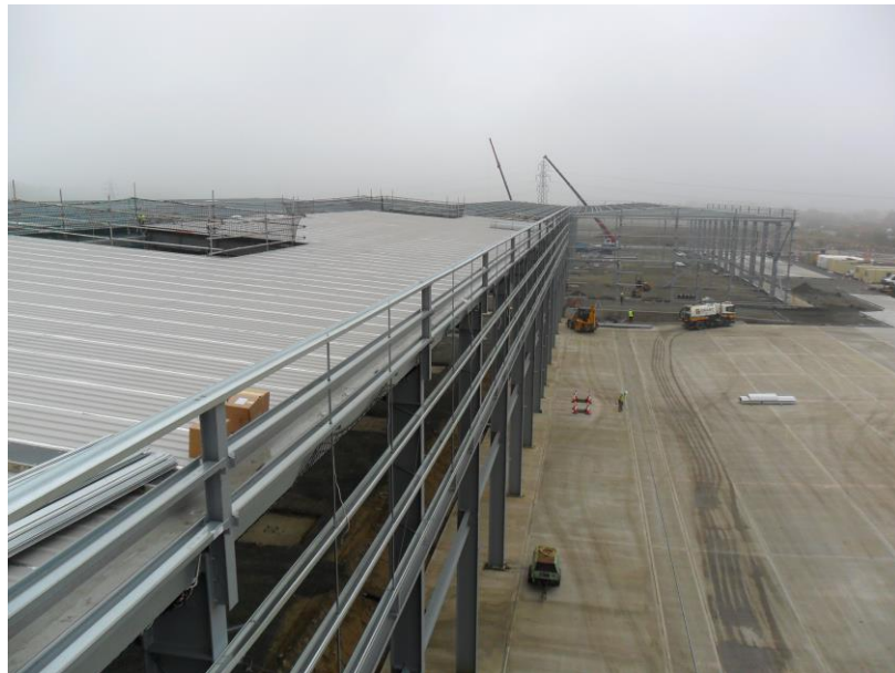
Image 4: Primary and secondary steelwork properly installed
