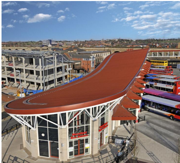
Mansfield Bus Station. Image courtesy of Kalzip Limited
