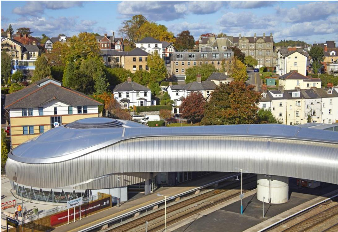
Over 1,000 individual Kalzip aluminium standing seam sheets have been installed on Network Rail's stunningly designed new station at Newport, South Wales. As well as straight, tapered and smooth curved Kalzip sheets, many revolutionary Kalzip XT profile sheets of various shapes and sizes were used for significant parts of the link footbridge and concourse buildings where the aluminium cladding is curved both on plan and in section.
