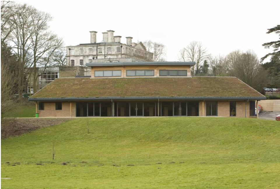
A green roof on Kingston Maurward College, Dorset - image courtesy of Euroclad
