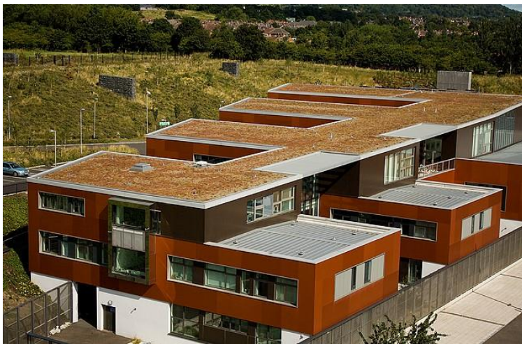
A Kalzip green roof at Grove Wellbeing Centre, Belfast
