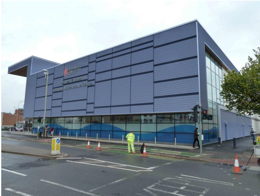
Roll formed louvre profile and live louvre cladding were specified for the Queen Elizabeth Diamond Jubilee leisure centre at De Montfort University, Leicester. Image courtesy of Architectural Profiles Limited
