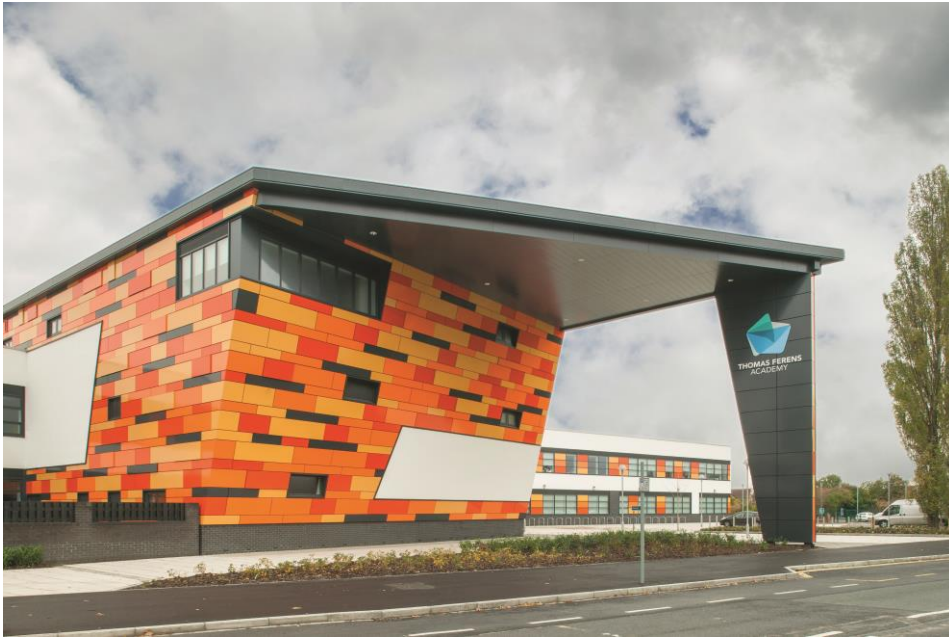
The AshTech rainscreen cladding system was specified at the Thomas Ferens Academy, Kingston upon Hull. Image courtesy of Ash & Lacy Building Systems Limited
