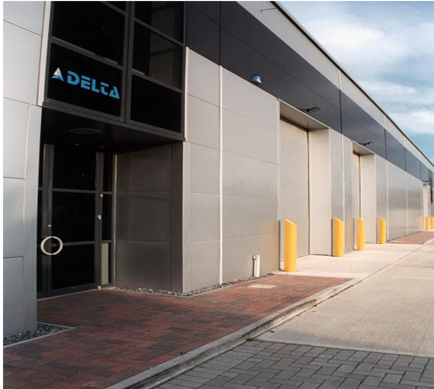
Tritherm composite panels on the Harlow business park. Photo courtesy of Architectural Profiles Limited
