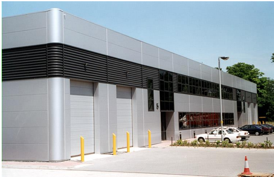
Tritherm composite panels on the Nimbus business park. Photo courtesy of Architectural Profiles Limited
