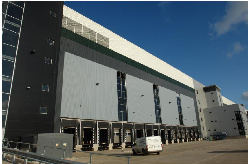
SolarWall was specified at Marks & Spencer, Castle Donington
