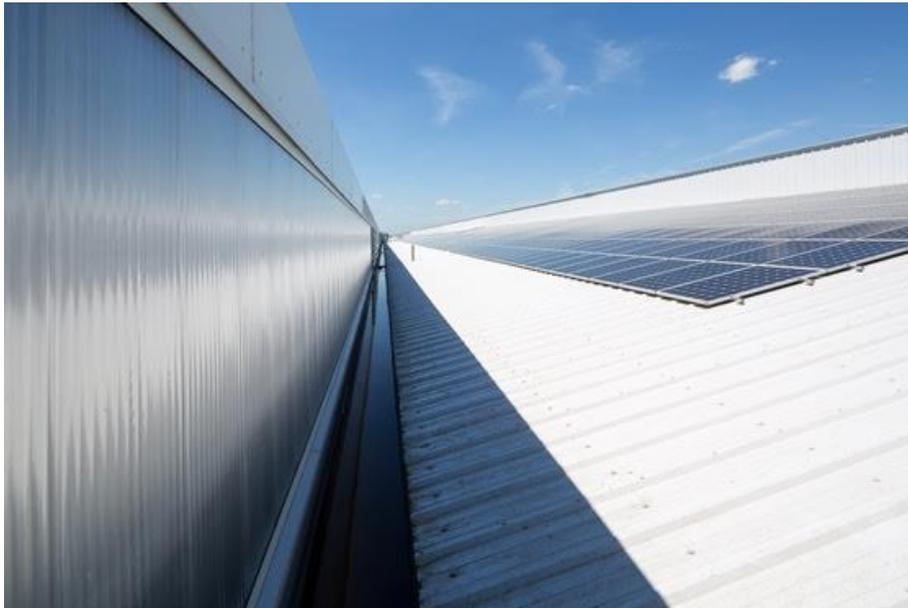
*The Marlon Clickfix interlocking glazing panels simply clicked together to create the seamless northlights.*
