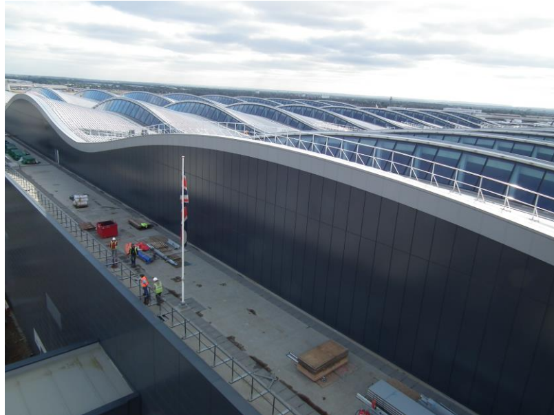
Construction phase of Terminal T2A Heathrow
