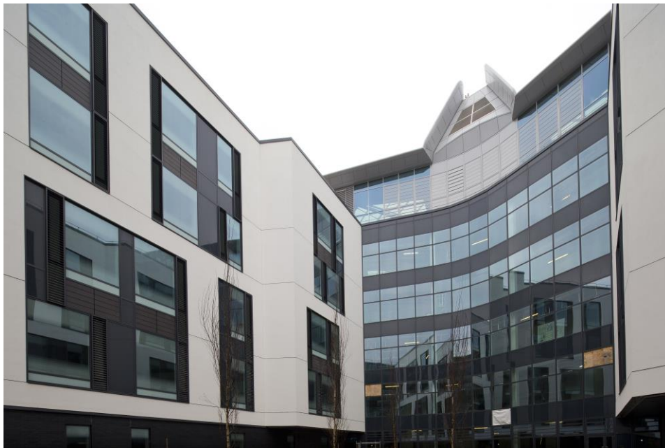
Southmead Hospital, Bristol. Courtesy of Euroclad Limited
