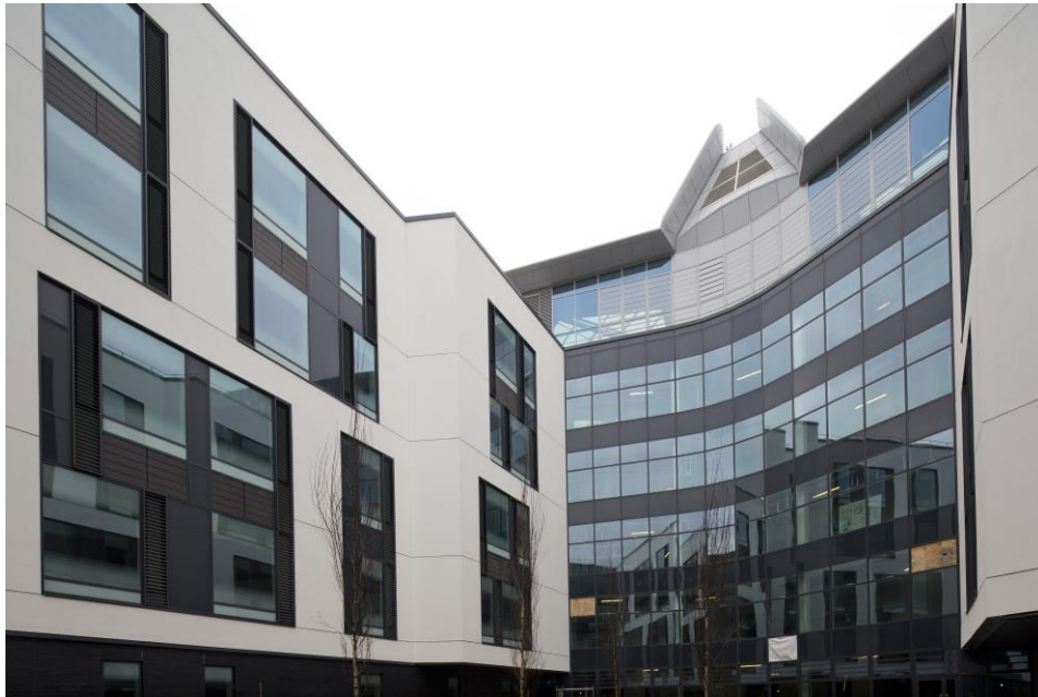
Southmead Hospital, Bristol. Courtesy of Euroclad Limited
