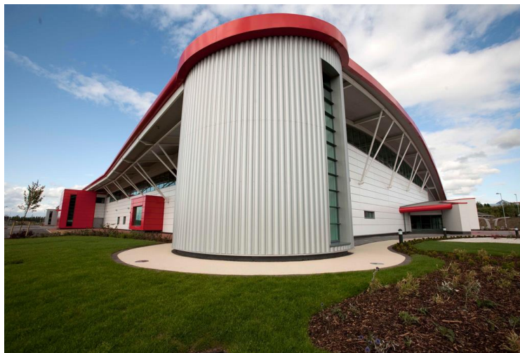
Vodafone contact centre, Stoke on Trent. Image courtesy of Euroclad
