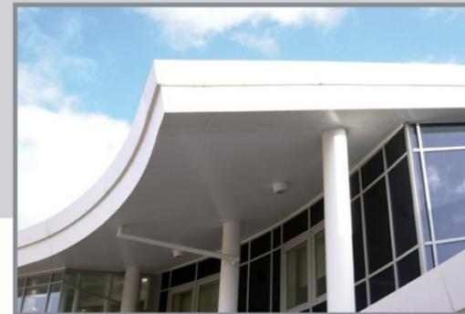
Fascias are used on vertical faces and soffits for the underside of horizontal faces. These items are often treated as cladding, however they are mentioned here because they are often used to create architectural features to complement or contrast with the main cladding system.
