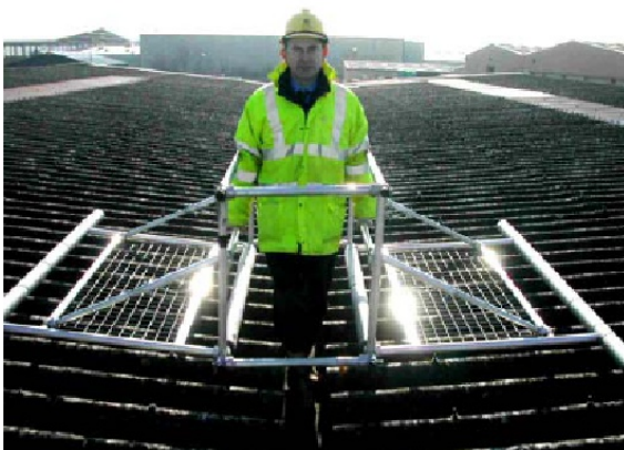
Figure 12 valley gutter protection
