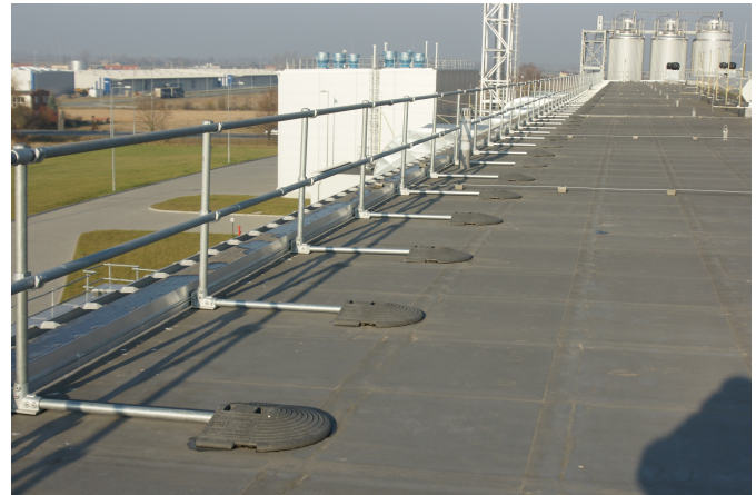
Figure 7 Parapet edge protection using tube and fitting
