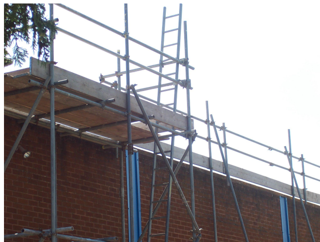
Figure 3: Ground Supported Edge Protection
