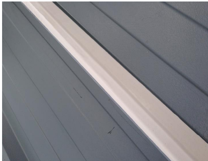
Airtightness sealing with liner panel tape
